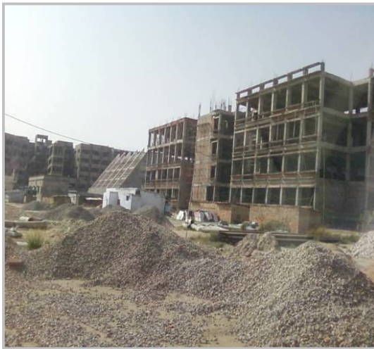
Hospital and Admin Block
