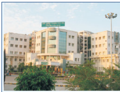
Hospital Block of RIMS, Safai
